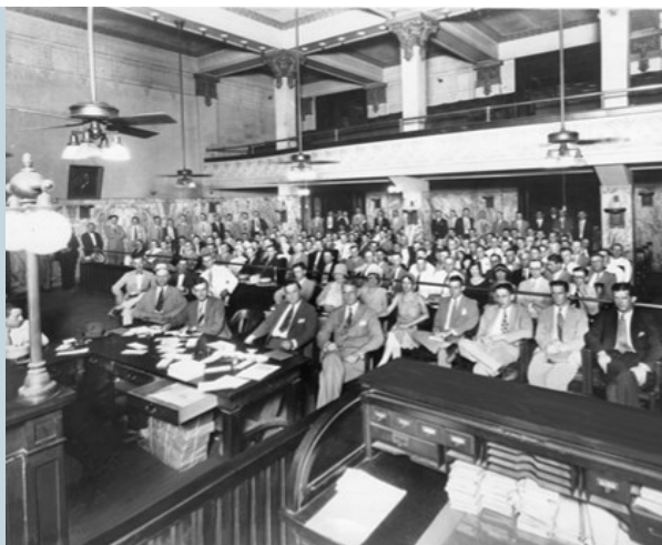
The north courtroom of the 1910 Courthouse in 1920.
